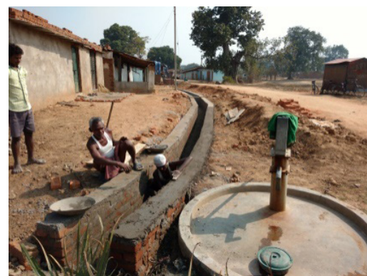
Drain Constructed under 14th FC
